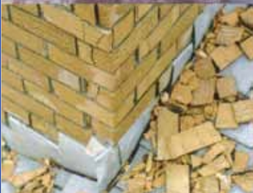
Water penetration and freeze/thaw damage result in loss of insulation value and lead to structural failure.
