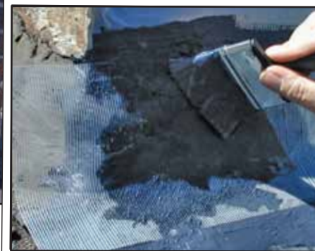
For added strength and flexibility, a fiberglass fabric is embedded between 2 coats of FlashSeal Elastomeric Sealant
