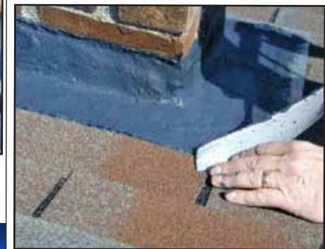
In most cases the roof deck and chimney are taped off to produce a neat appearance of the finished application
