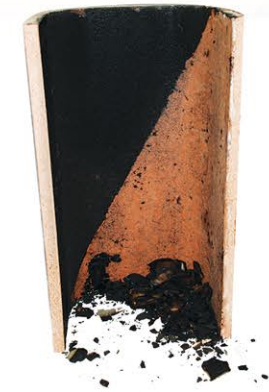
Creosote falls off easily as PCR dries
